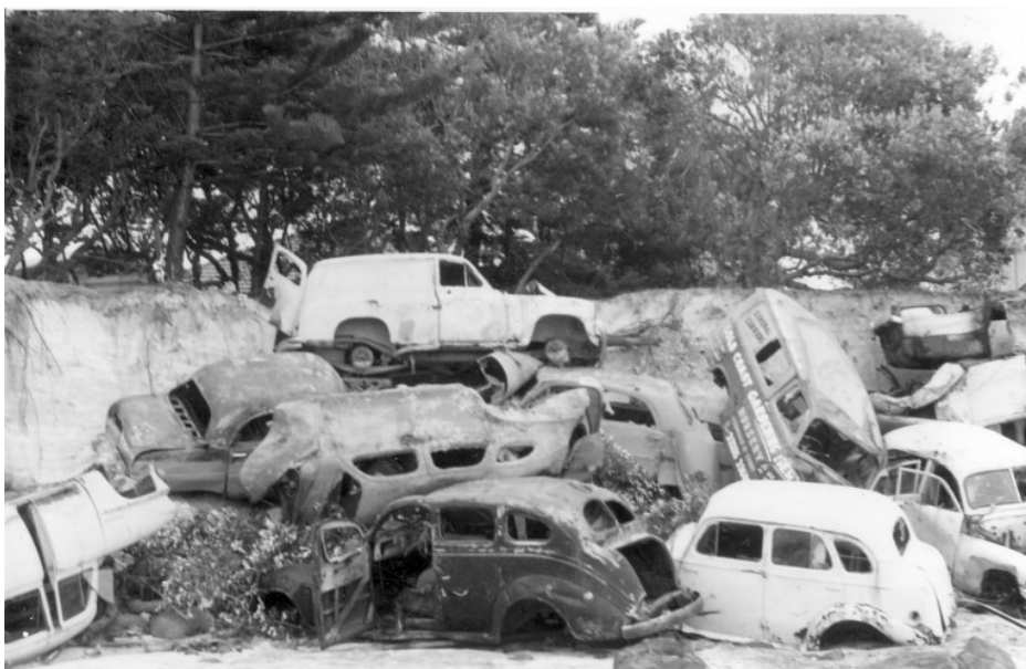
Figure 4 1967 Use of old car bodies for coastal protection Gold Coast style Source: GCCM (2013)
